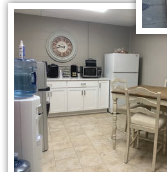
Renovated the employee kitchen and bathrooms
